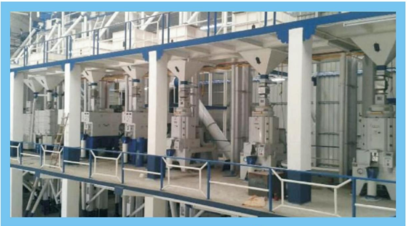
RICE MILL PLANT
